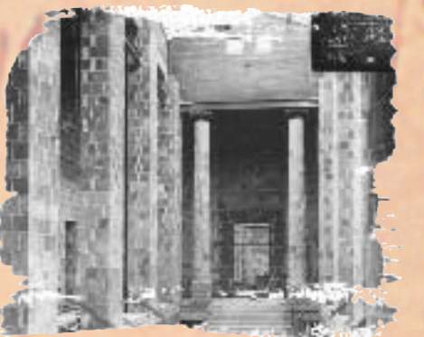
Interior under construction, first floor, north end, 1910.
