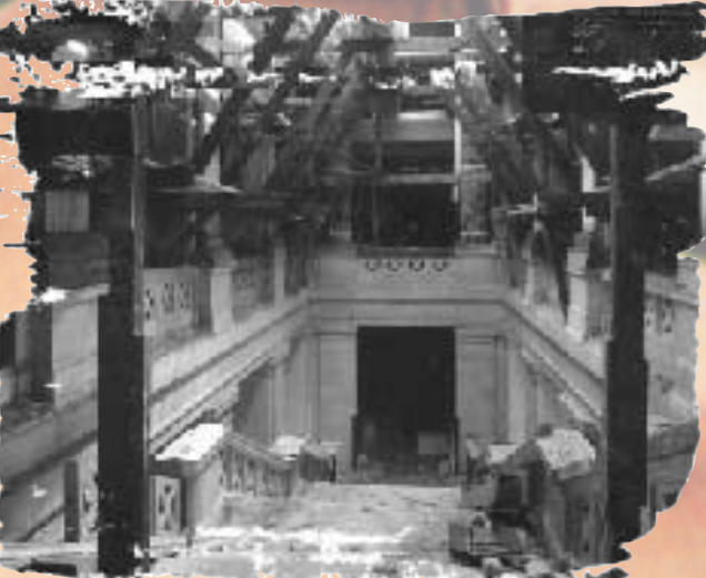
Interior under construction, third floor looking south, 1910.
